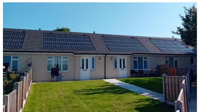
Figure 6 – Tyddyn To, Menai Bridge
